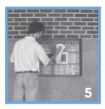
When the mortar begins to set, remove the wedges, fill the holes, smooth the joints with a trowel and clean the glass with a cloth.
