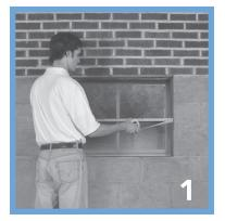
To make sure your new window will fit properly, measure the window opening as if the frame were already removed. You will need a space of approximately 1/4" to 1" all the way around the perimeter for mortar.
