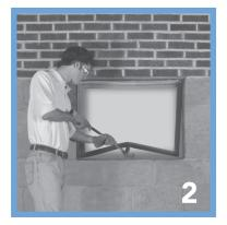
Remove the window sash and then remove the window frame by bending the top and bottom in toward the center or by cutting it. Remove the old mortar sill if necessary.
