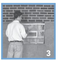
Set the new window into place on top of 2 wedges, check that it is plum and level, then secure it with 2 wedges at the top. If you are installing a vented window, the vent latch should be located on the inside at the top.
