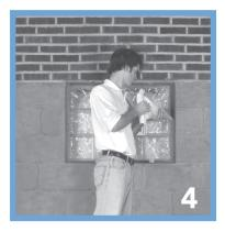
Mix the mortar according to the instructions on the bag. Apply the mortar around the perimeter using a grout bag or a trowel. Make sure the joints are completely full.
