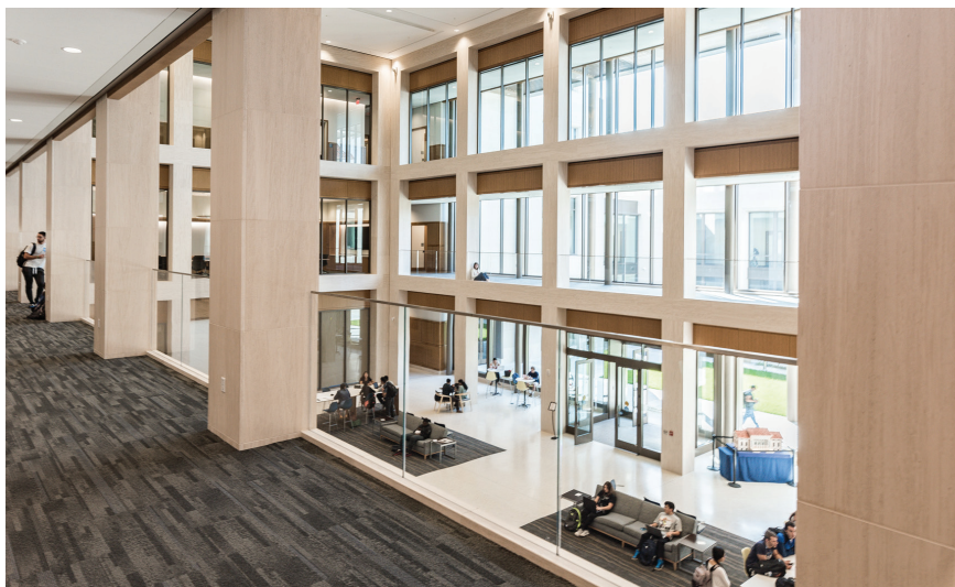
Take it inside. Thinner stone allows for interior applications and keeps the load on the wall lighter.
